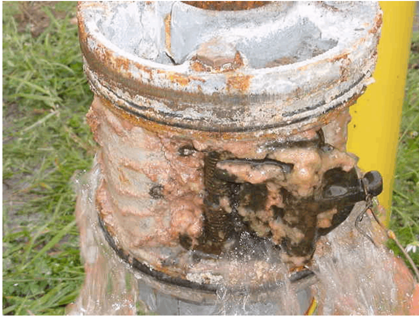
Example of Biofouling on a Pitless adapter
