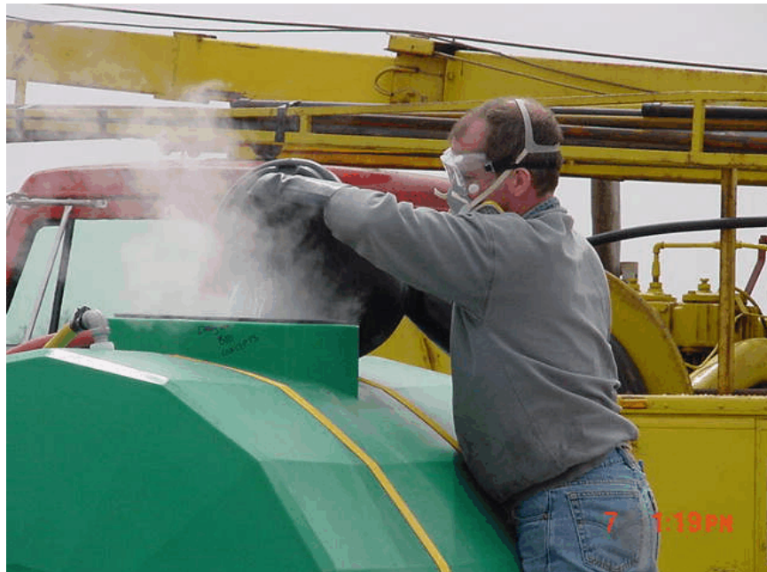
Chemicals being mixed with water used in treating the well
