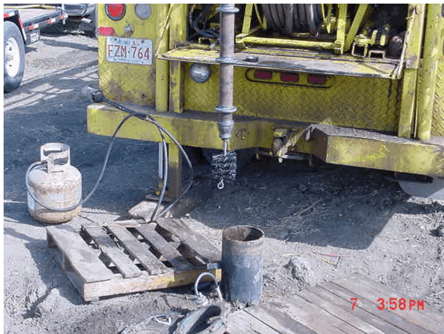
Cable rig setup with wire brush to scrape inside well casing
