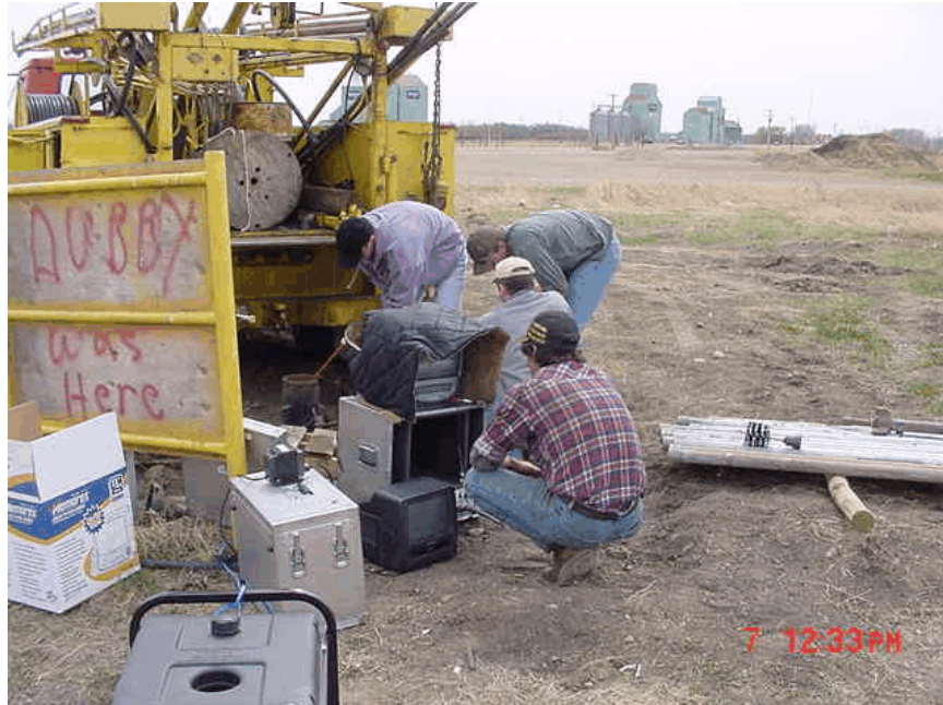
Video Inspection of the Well (done before & after treatment)
