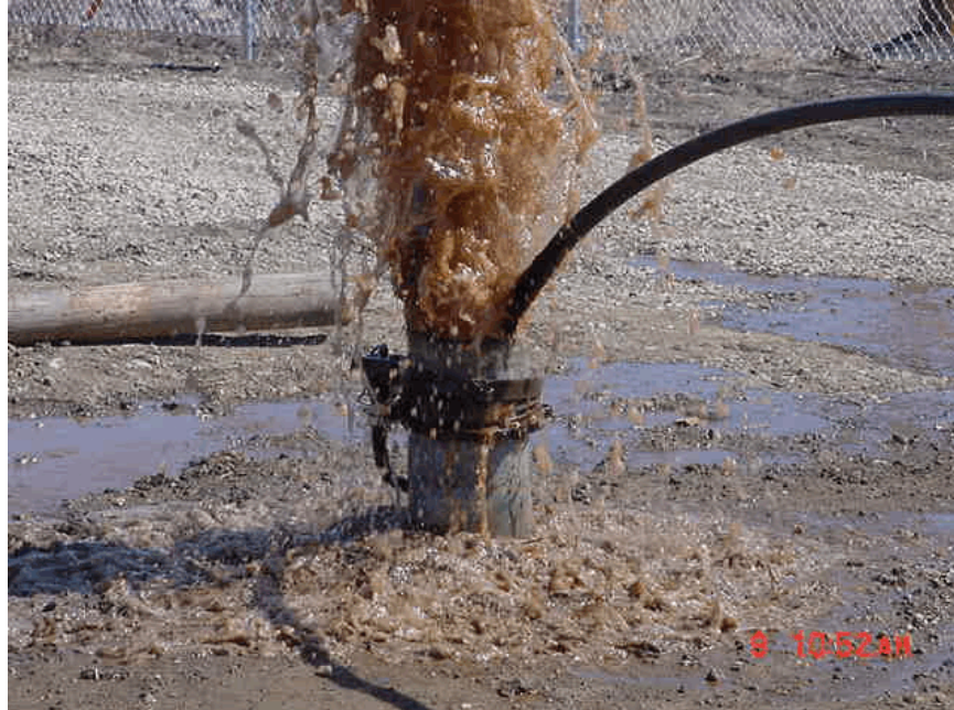
Blowing out well after primary treatment
